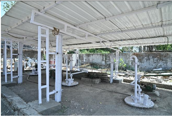
Underground storage tanks
